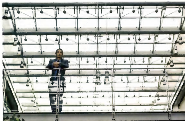
Air conditioning use can be reduced by the use of window film
