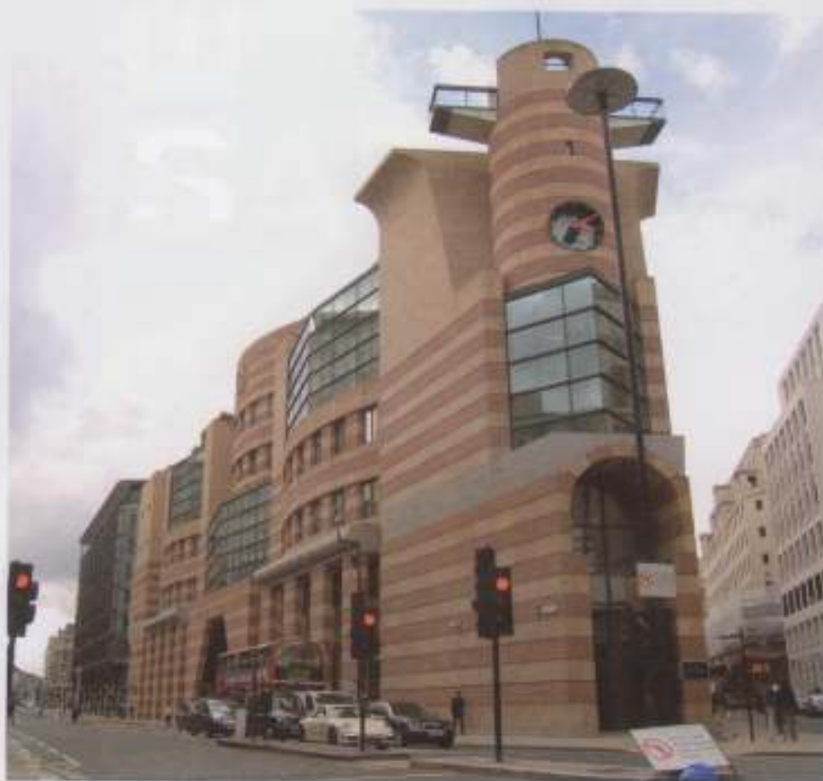
Number 1 Poultry, London, is protected with Solar Gard Armorcoat 7 mil Clear Safety Film
