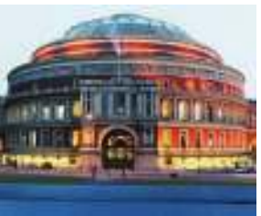
The Royal Albert Hall has installed Armorcoat, an innovative product by Bekaert
